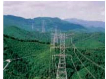
Ohkawachi power lines (500,000 V) (Kansai Electric Power Co.)
