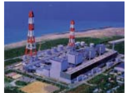
Atsumi Thermal Power Station (Chubu Electric Power Co.)
